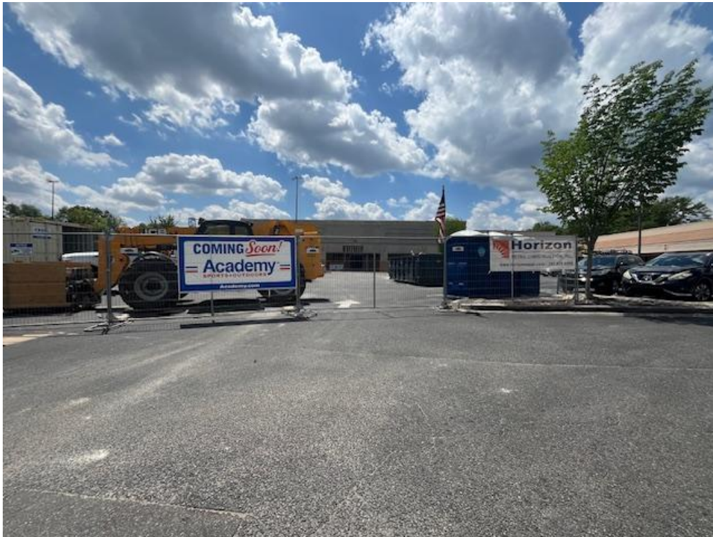
Subject Property: view of the property from the parking lot along the ROW on East Northside Drive, facing west.
